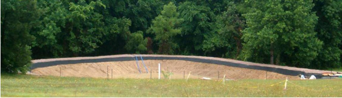
The final size of our pond is 100' long by 60' wide. Outside the pond area, the contractor found a natural spring and dug a well. We set up a submersible pump inside the well with an external on/off switch and piping to the pond.
